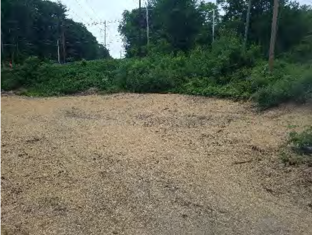
Fig 5: Dewatering basin location at Str. 32. Basin removed and restored. Viewing south. (06-11-20).
