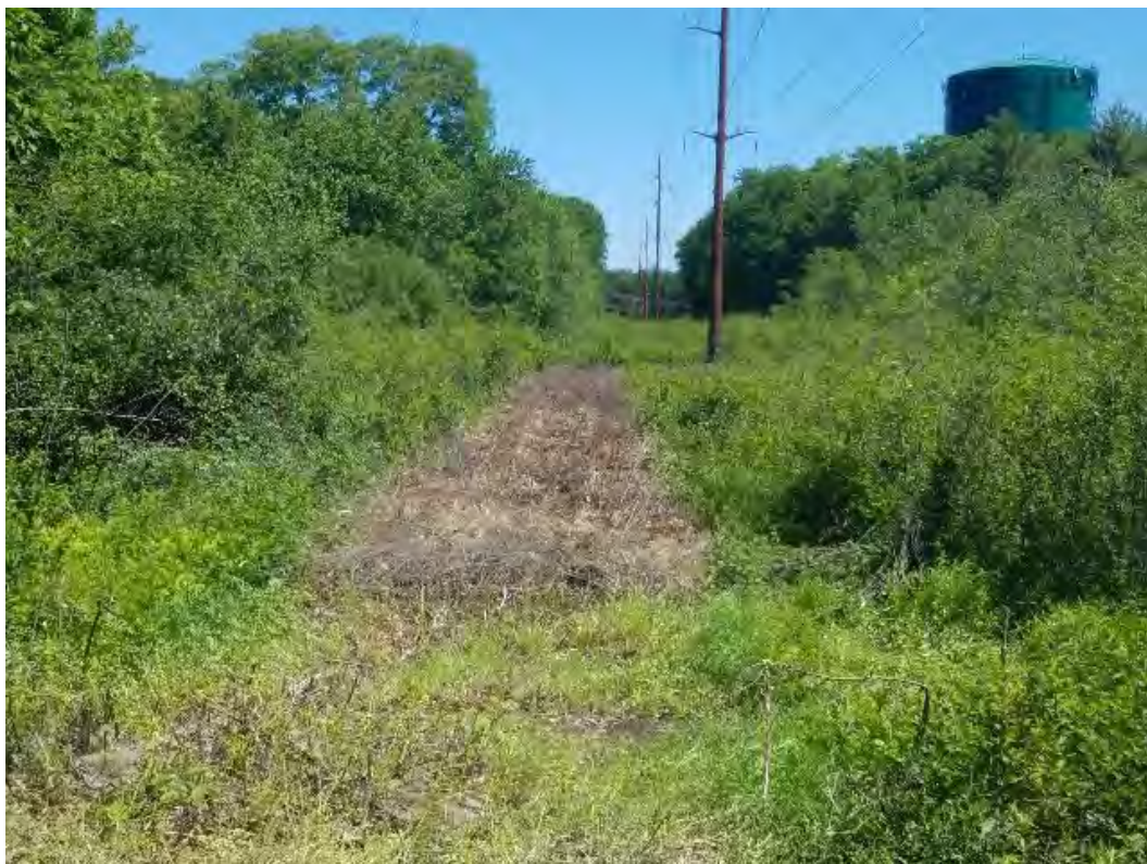
Fig 20: Access road to Str. 35, through wetland DW41 restored. Viewing north. (06-17-20).
