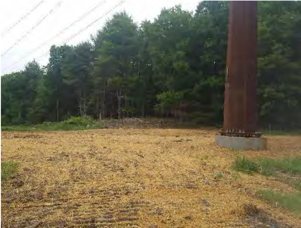
Fig 3: Str. 85 work area restored. Viewing northwest. (06-11-20).
