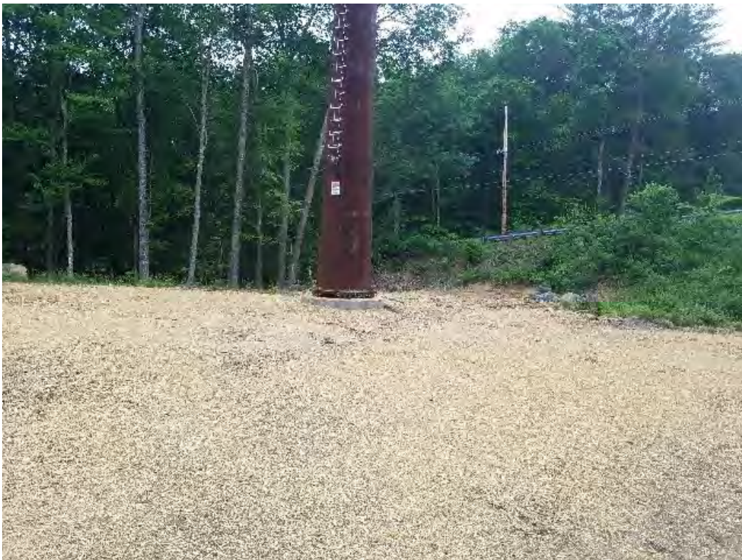
Fig 6: Str.32 work area restored. Viewing southeast. (06-11-20).
