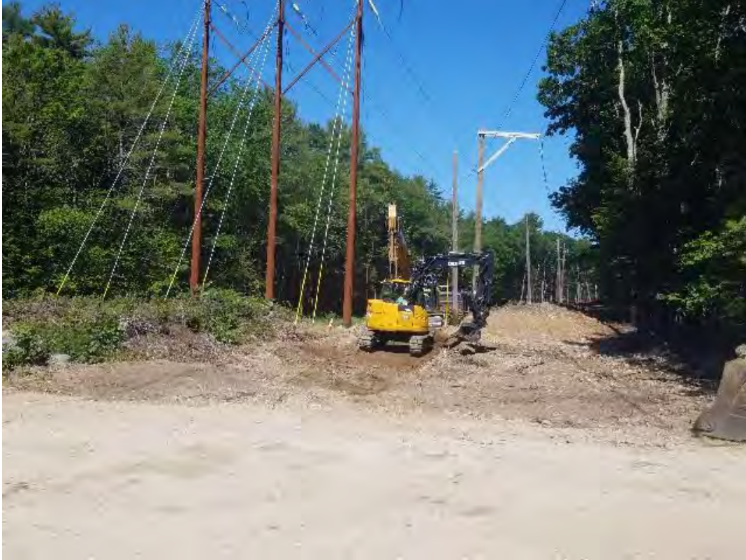
Fig 19: Crew beginning to remove access road to Str. 98. Viewing west. (06-17-20).
