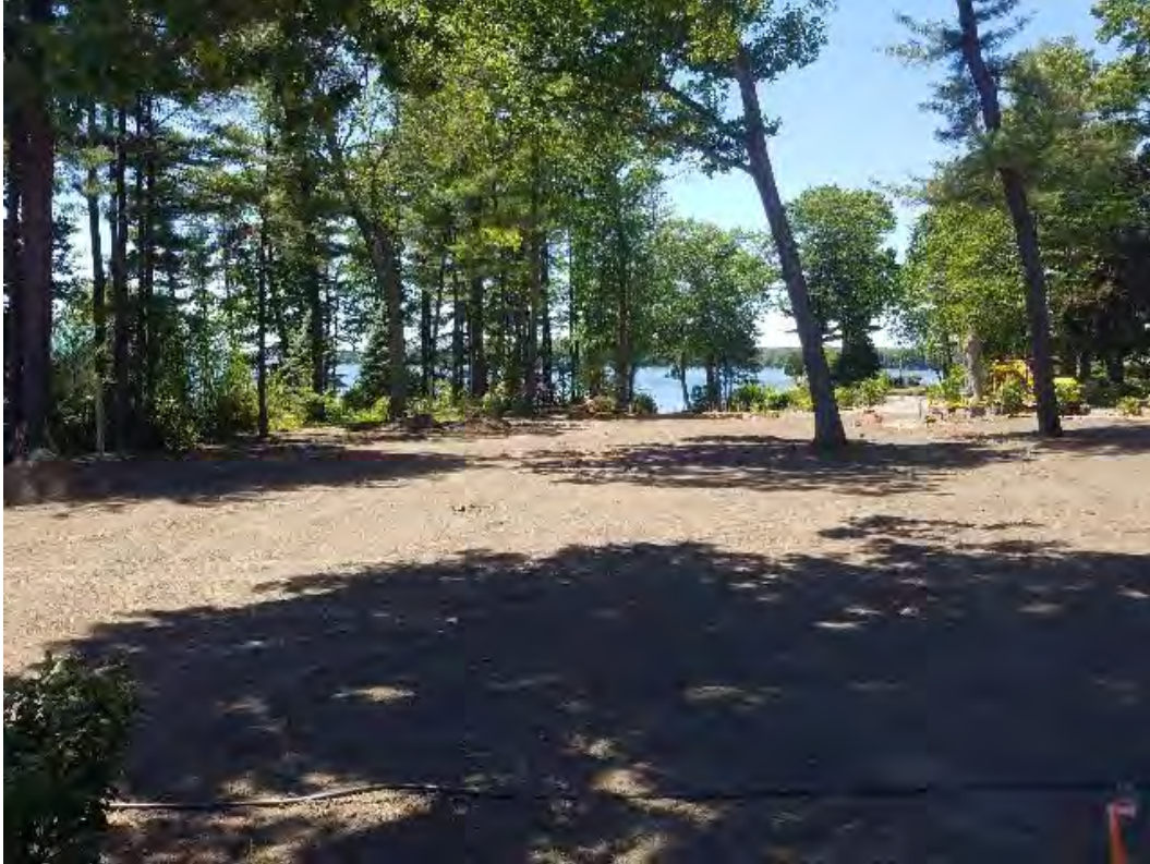
Fig 15: Landscape activities at Gundalow landing/east side of the Bay. Viewing west. (06-16-20).
