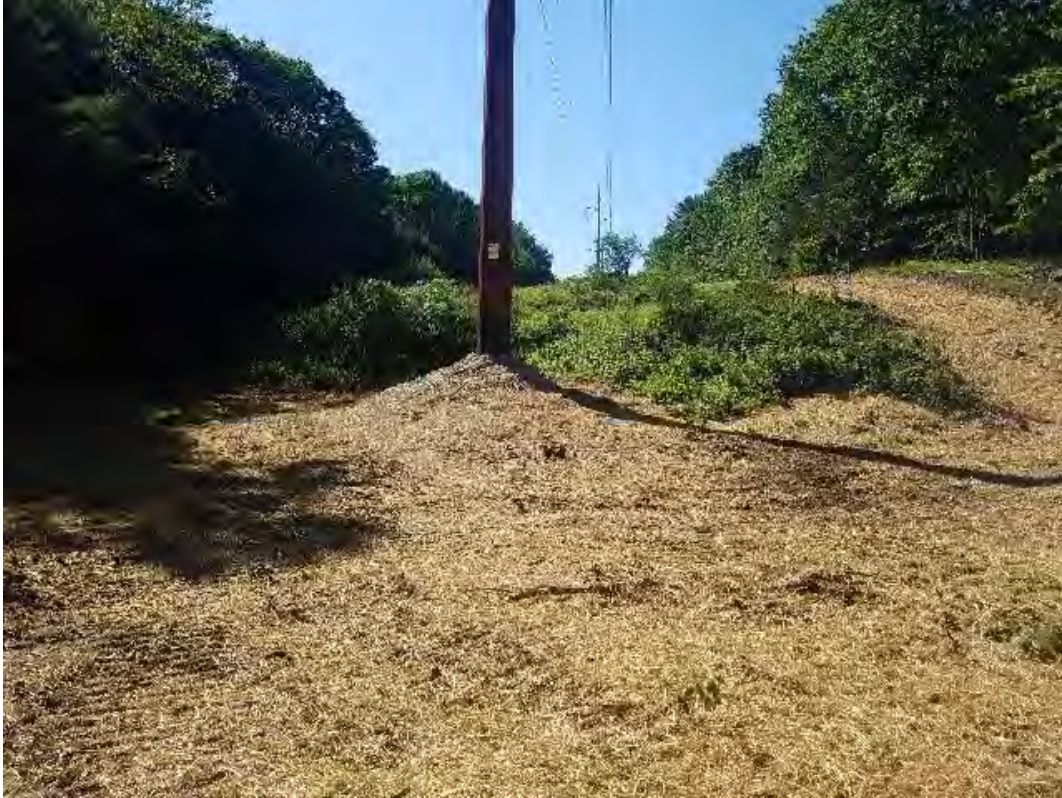
Fig 9: Str. 86 work area restored. Viewing south. (06-16-20).
