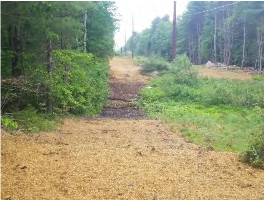
Fig 4: Access road between Strs. 85-84, through wetland DW30 restored. Viewing west. (06-11-20).
